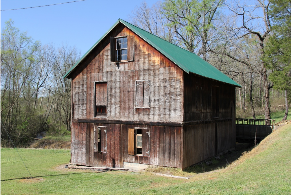
McKinney Mill, east elevation, view to southwest
