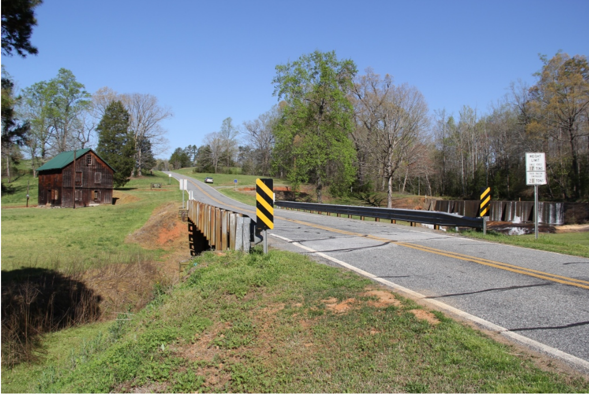
Bridge No. 88, view to northwest along McKinney Mill Road (SR 1793)
