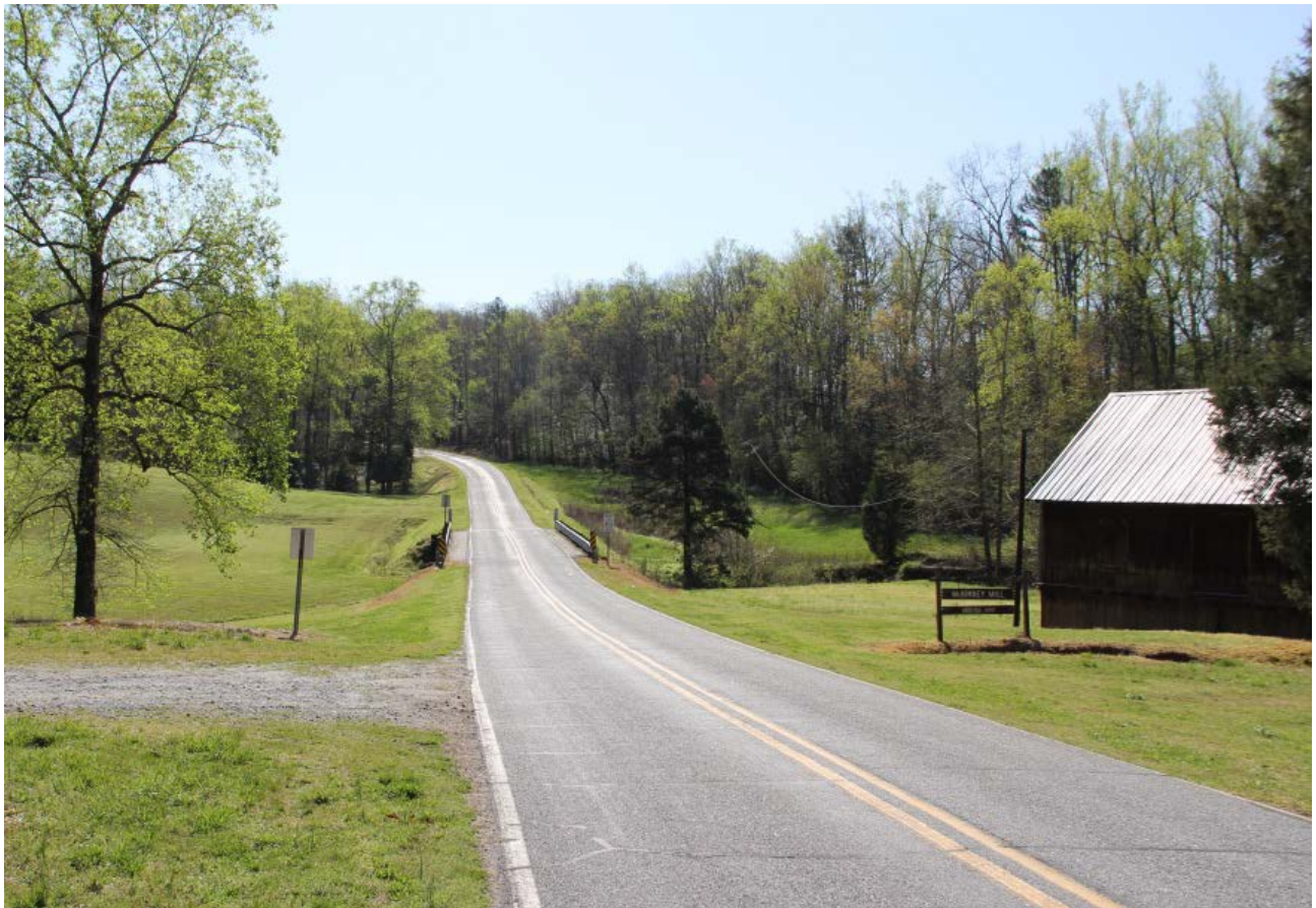
Bridge No. 88, view to southeast along McKinney Mill Road (SR 1793)
