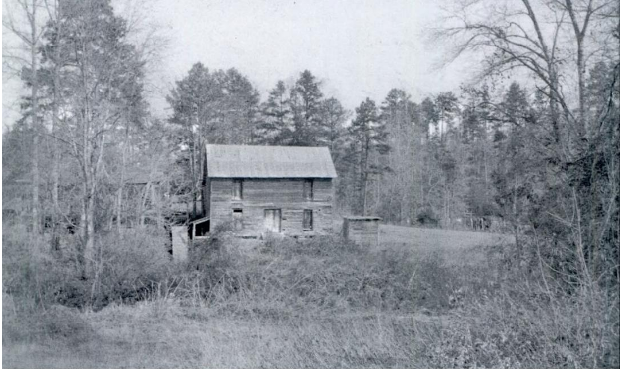
McKinney Mill, date of photo unknown [Source: Colfax Township (2011), 49]
