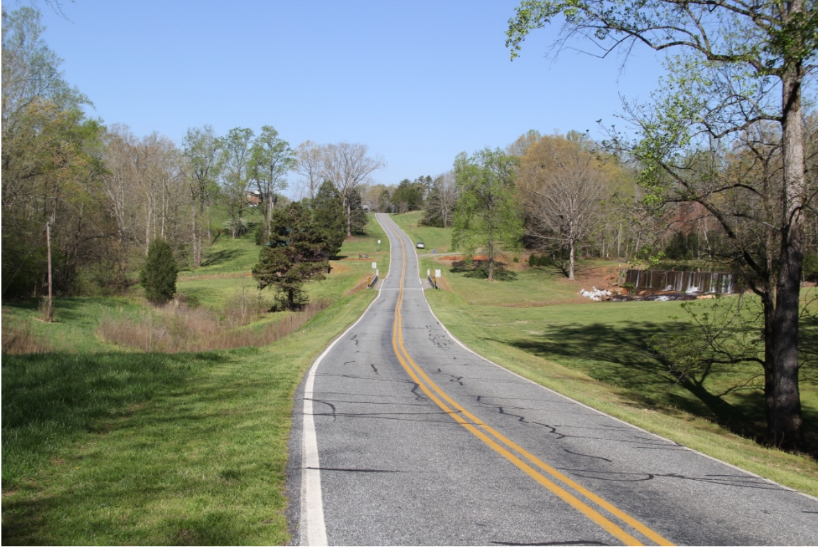
View to northwest along McKinney Mill Road (SR 1793)
