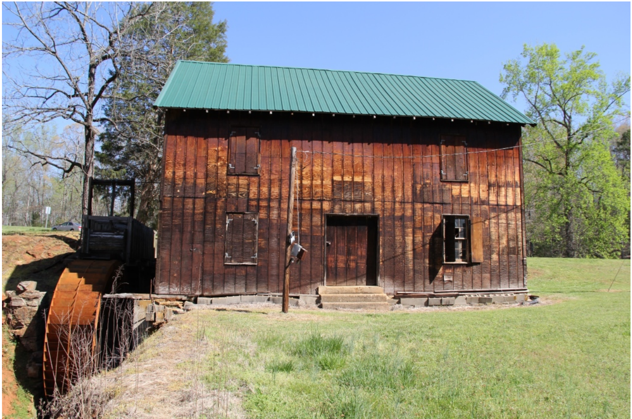
McKinney Mill (RF 52), 926 McKinney Mill Road, façade, view to north
