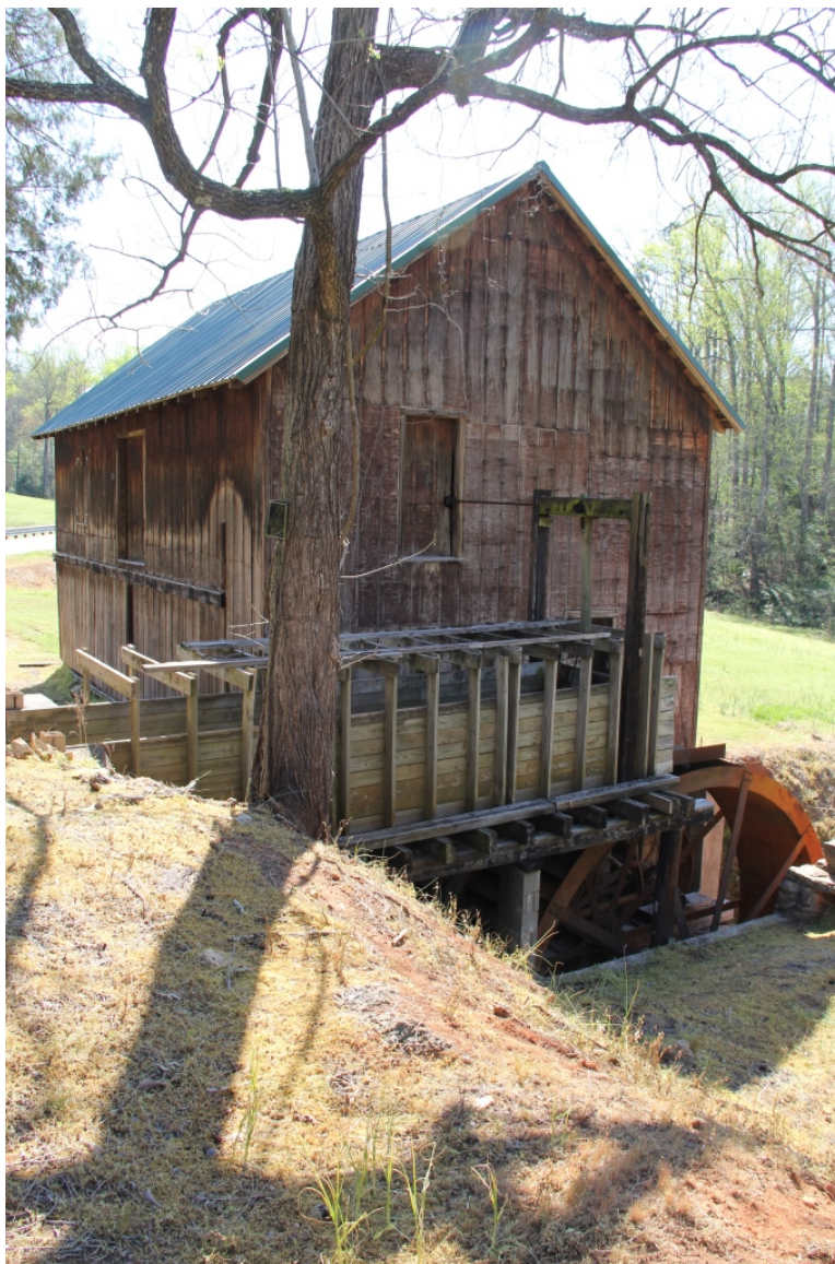
McKinney Mill, west elevation, view to southeast
