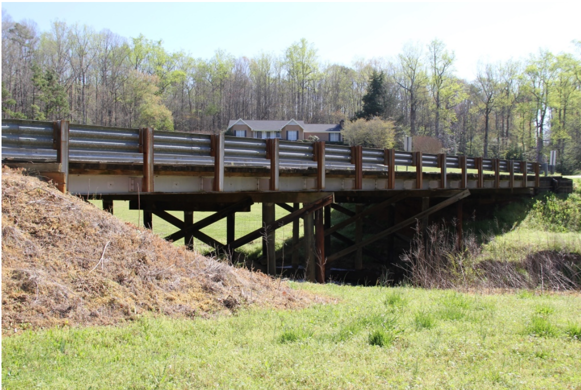
Bridge No. 88, oblique view to northeast
