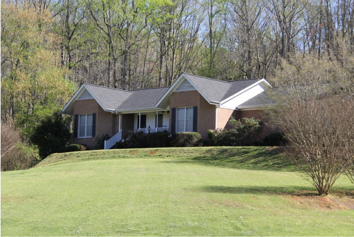
Ivey Ray and Mary Evelyn Mauney House, 991 McKinney Mill, oblique view to north
